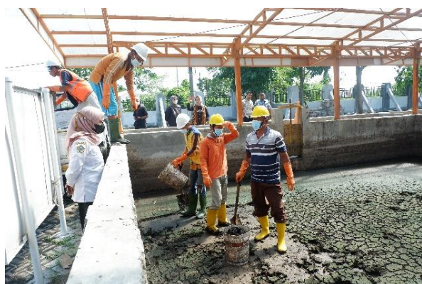
UPTD PLCD Gresik workers harvesting dry fecal sludge at the Betoयोगुci IPLT.
